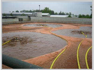
FBC Technologies, Inc. brought in a 44HP system to replace the 100HP of splashers running at the plant. **This is better than a 2:1 HP replacement ratio!** The single positive displacement blower feeds a valved manifold that individually controls flow to each of the units. The client was interested in maintaining a certain level of residual dissolved oxygen in the tanks at all times using the O<sup>2</sup>ctopus
