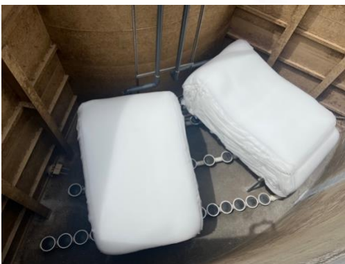
WavTex Modules Upon Installation in Aerated Tank, before tank is refilled
