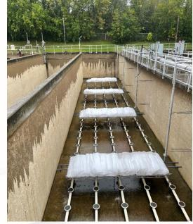
Left: WavTex modules installed over fine bubble aeration
