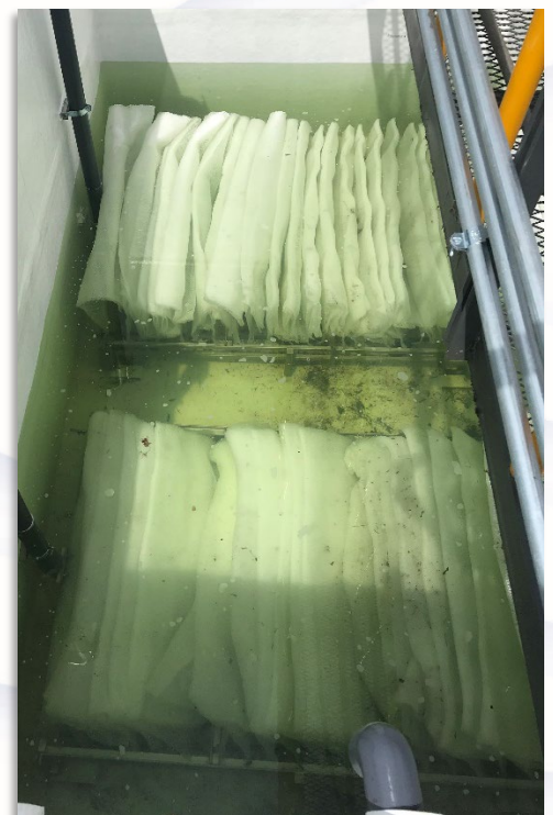
Bottom Right: WavTex modules in tank as it is being filled. The buoyant EnTextile sheets are beginning to stand.
