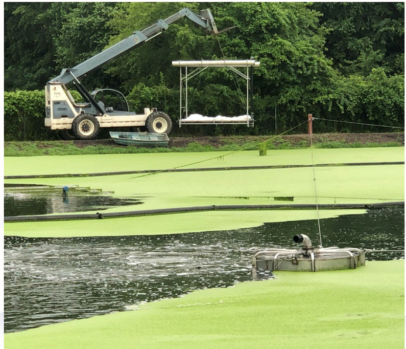
Background: WavTex module being installed via lift truck Foreground: Octopus module in lagoon
