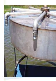
Octopus is a flexible floating fine bubble diffuser system
