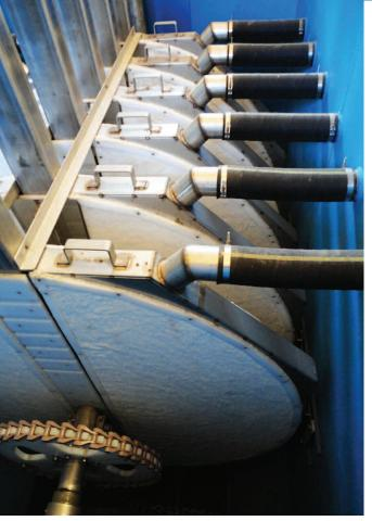
FlowTex is a user friendly, tertiary disc filter suitable for both small and large flow applications. The patented FlowTex filter with outside-to-inside flow incorporates a fixed disc with a rotating vacuum head for backwashing. The vacuum assembly is designed to keep from touching the cloth media. This provides for extended cloth media life.
