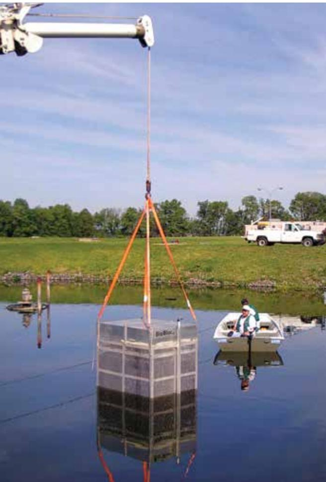
*BioBloc units float into place as the system is secured between stainless steel cables that extend from shore to shore.*
