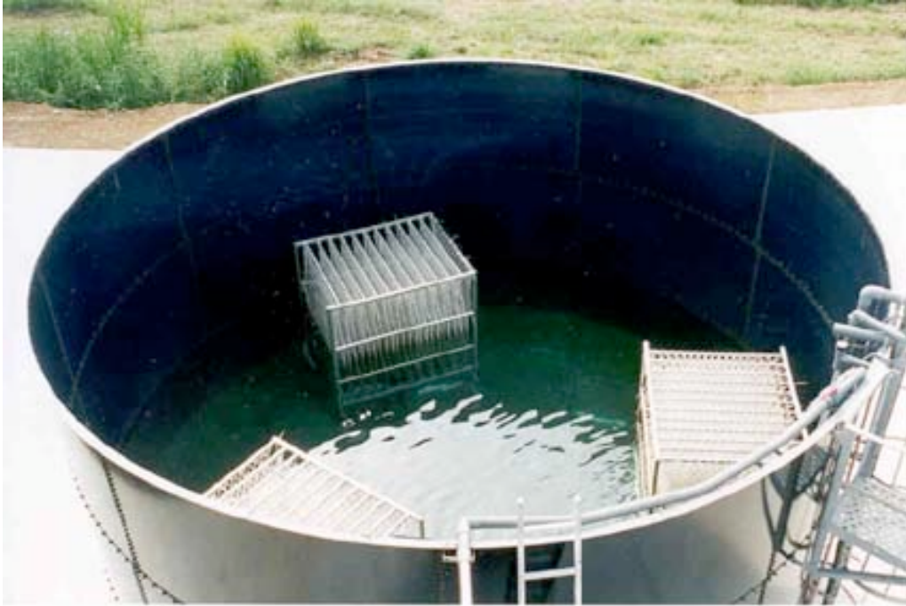
Figure 3: Close up of the BioWeb fixed-film media
