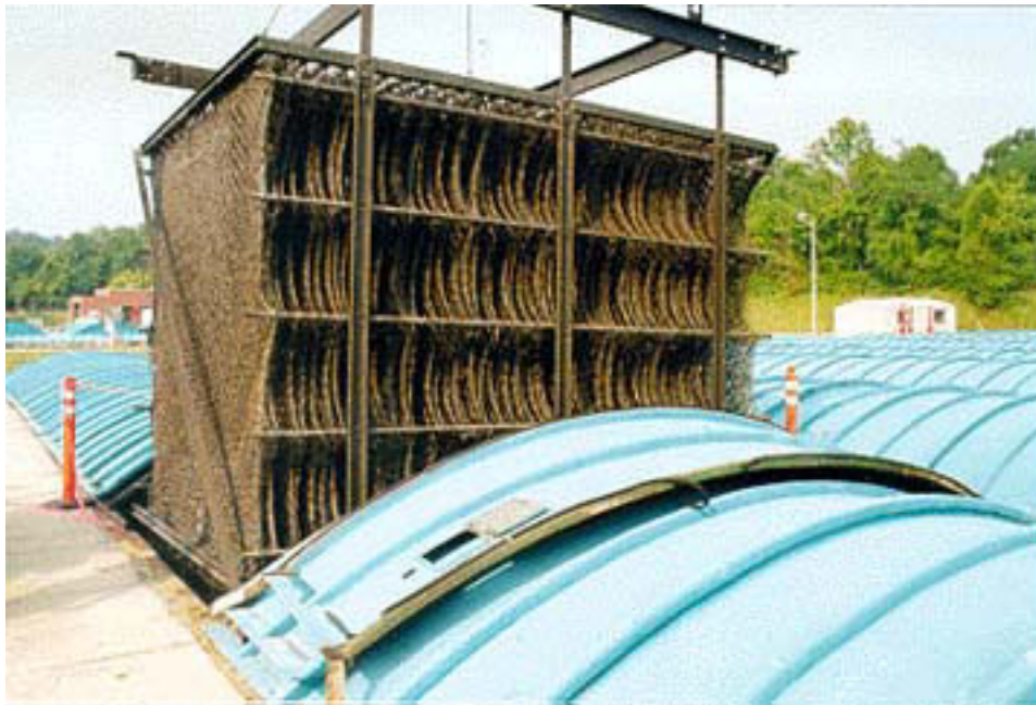
Figure 3: BioWeb frame with attached biomass after several months of operation
