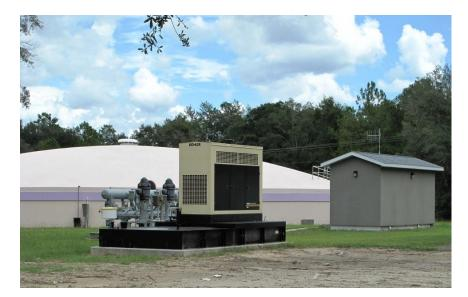
**Figure 3.** Precon One MG Ground Storage Tank with High-Level Disinfection using Sodium Hypochlorite.
