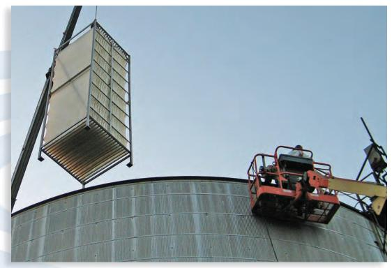
Media Installed 15 Webitat modules with over 127,040 ft<sup>2</sup> of BioWeb media
