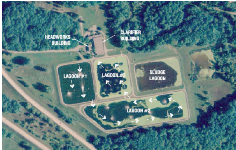
Figure 1: City of Clare WWTF
