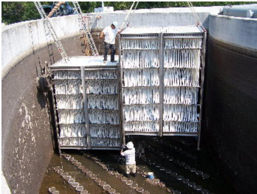
Webitat is a new, next generation BioWeb™ IFAS system engineered to actively manage the attached biomass environment. Shrouding the four vertical sides of the module and providing dedicated air supply underneath substantially enhances mixing and ensures a thin-film biomass. The enclosed Webitat module with its controlled biofilm thickness is a high-rate biological reactor.
